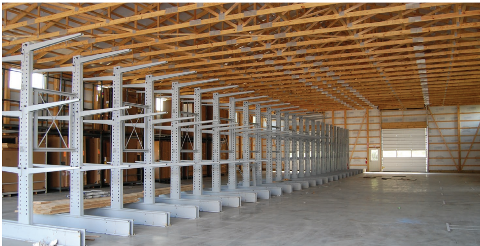
Racks will be used to store doors, windows and building materials
