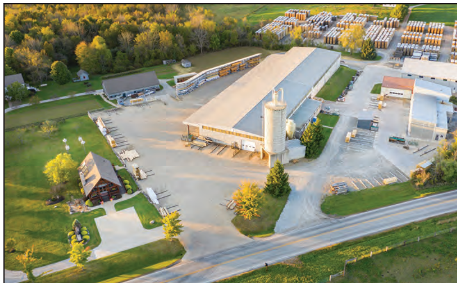
The Hochstetler complex includes the Black Fork model (lower left), the mill (center), the dry kilns (upper right) and air-drying yard (far upper right corner).
