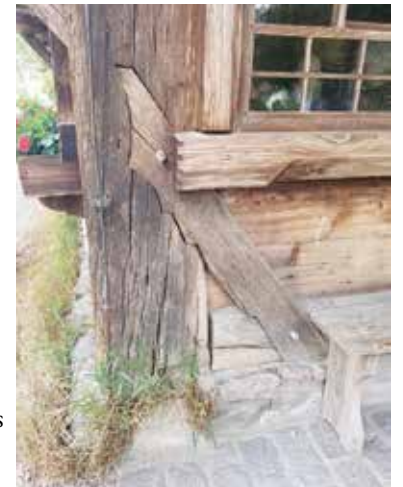
“Vogtsbauernhof” circa 1613 in Gutach, Germany. Intricate joinery overlays blockwork infill.
