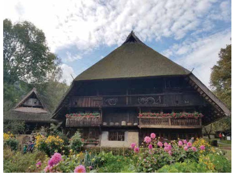
"Vogtsbauernhof" circa 1612 in Gutach, Germany. Combined livestock & living quarters. Reed thatched Dutch hip roof, mixture of blockwork and timber frame construction, original building at the museum.
